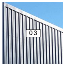
03 BROWNBUILT 900 02 (DIMOND ROOFING) VERTICAL
